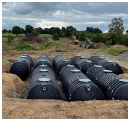
Installation of 862PE oneAdvanced, Dundrum House Hotel.
